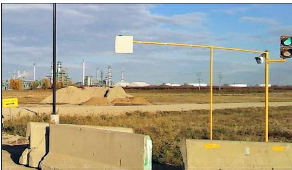
When a truck comes within range of the Times-7 reader antenna suspended overhead, a Feig Electronics reader captures the unique ID number encoded to its windshield tag. A traffic light installed beside the reader then turns green, signaling the driver to proceed.
